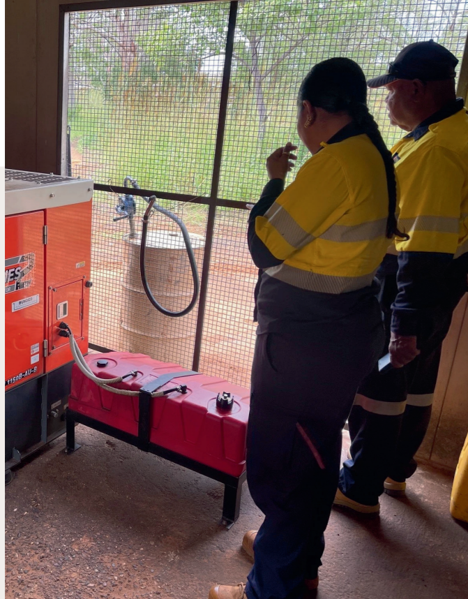
Terry Shadforth and Apprentice Power Worker Simone Long inspect existing power assets in a remote community
